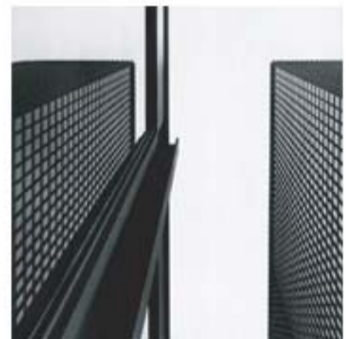
Twin Towers - 860 - 880 Lake Shore Drive, Chicago 1949 - 1951
