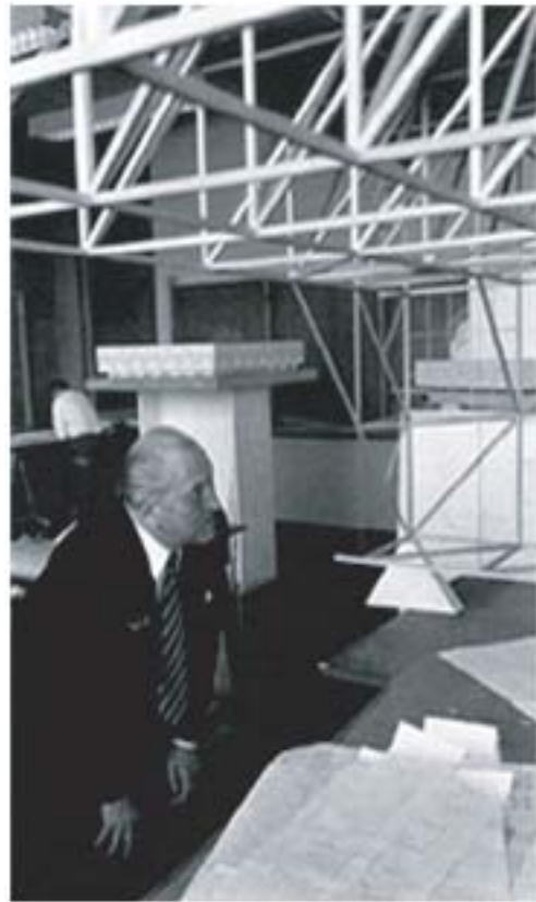
Inspecting the Chicago Convention Hall roof structure model
